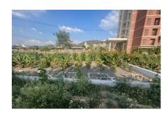
**Technology**: Anaerobic Baffle Reactor (ABR) + Constructed Wetland (CW) Capacity installed: 50 m<sup>3</sup>/d
